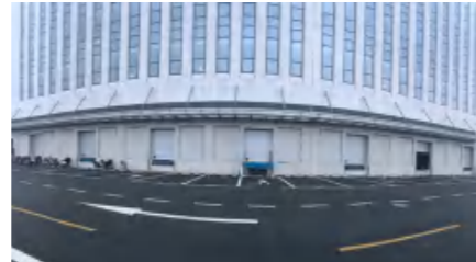
State Grid Zhejiang Electric Power Company
