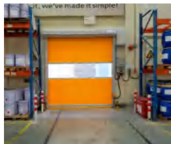
Explosion-proof door of chemical workshop
