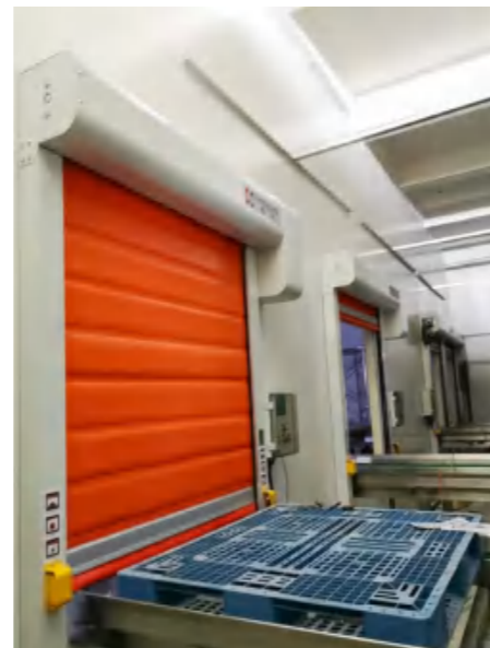
Insulation fast door of conveyor belt delivery port of pharmaceutical factory
