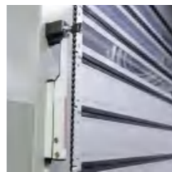
Power-off release manual device
